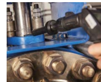
Testing a stem seal with 'live loading', using methane as the test medium and an FID leak detector.
